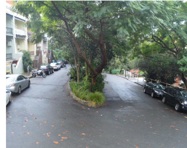
Figure 3 Hampden Street Median + Retaining wall. Showing level changes between upper and lower road existing retaining wall retains upper side of Hampden Street.
